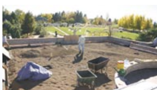
9 Light weight planting medium depth range from 4-12 inches.
