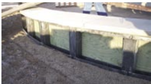
4 To keep wall lightweight, a rock veneer is utilized.
