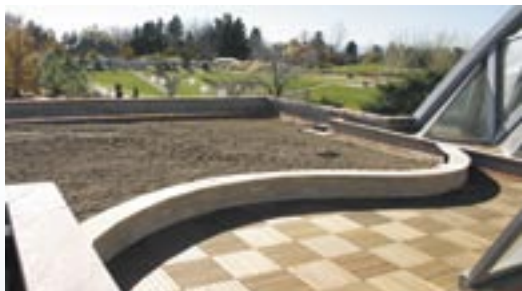
12 Deck is installed and green roof is ready for planting.
