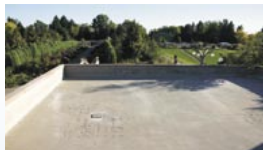
1 Starting with empty rooftop space, engineers determine structural weight capabilities.
