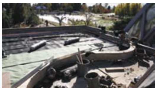
8 Moisture retention mat and drainage layer cover waterproof membrane.
