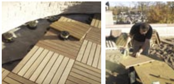
11 Installation of decking: View online videos for complete information.
