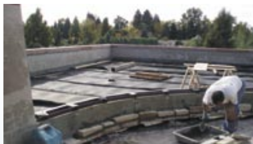
5 Rock wall is installed using sandstone rock & mortar.
